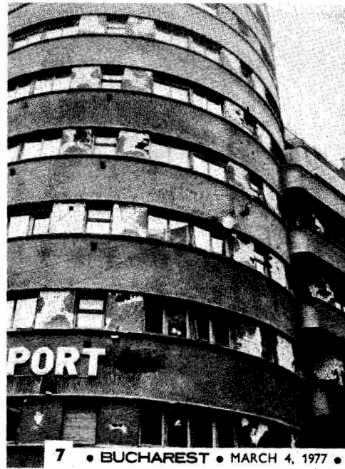
Cracking in exterior infill masonry walls of a reinforced concrete structure, erected before 1940
