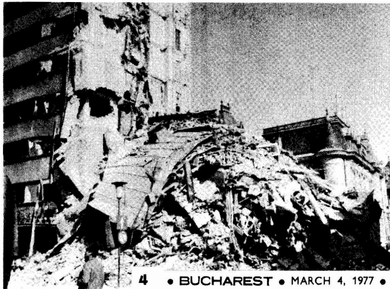
Complete collapse and wreckage of the multi-storey apartment building with reinforced concrete frames (erected before 1940)
